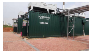
Figure 2 Biogas generator sets
