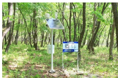
Figure 11 GIES ground station in Toudao Town
