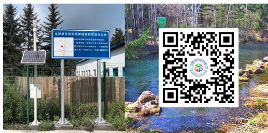
Figure 6 GIES ground station in Quanyang Town
